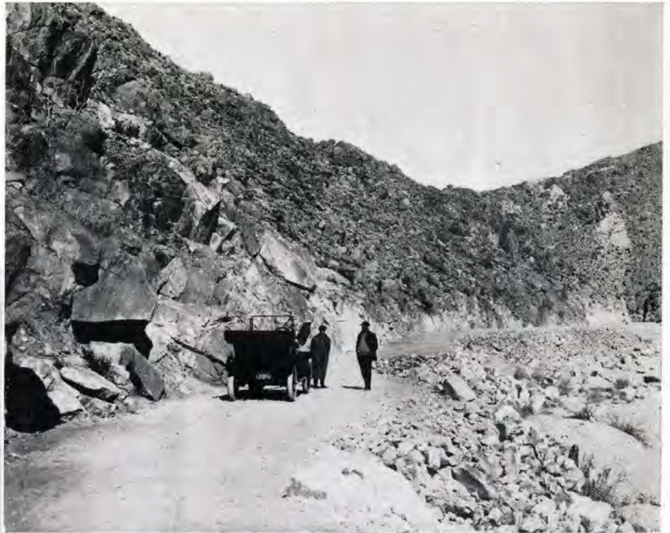
Before and After—Road Building in the Mountains Is No Simple Task, But It Can Be Done.
