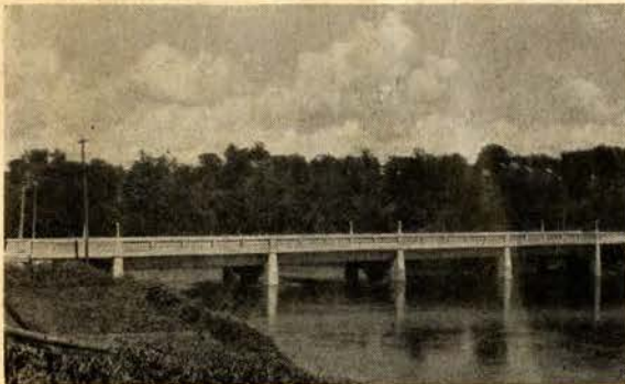
Bridge Over Clearwater River, Minn.
