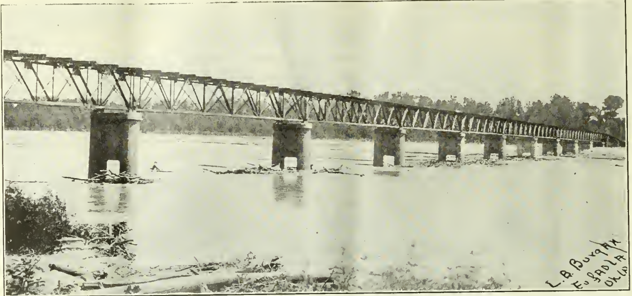
The Canadian River Bridge to be completed by May 15th. Slightly behind schedule but coming all right.
