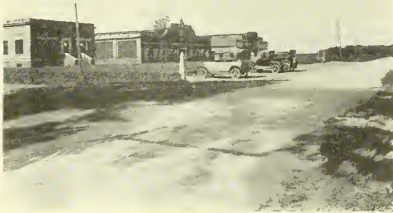
Hawkeye Supply Co. Plant, Front View.
