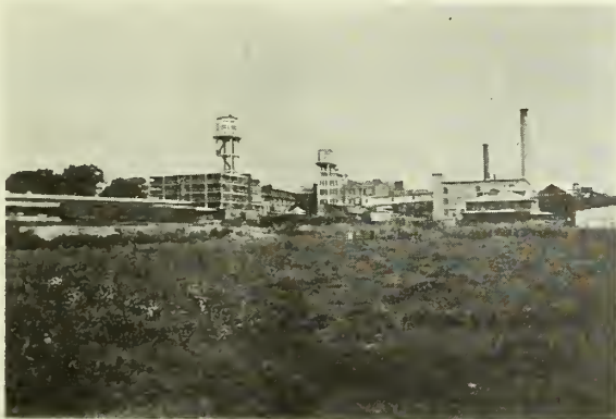
Mason City Packing Plant.
