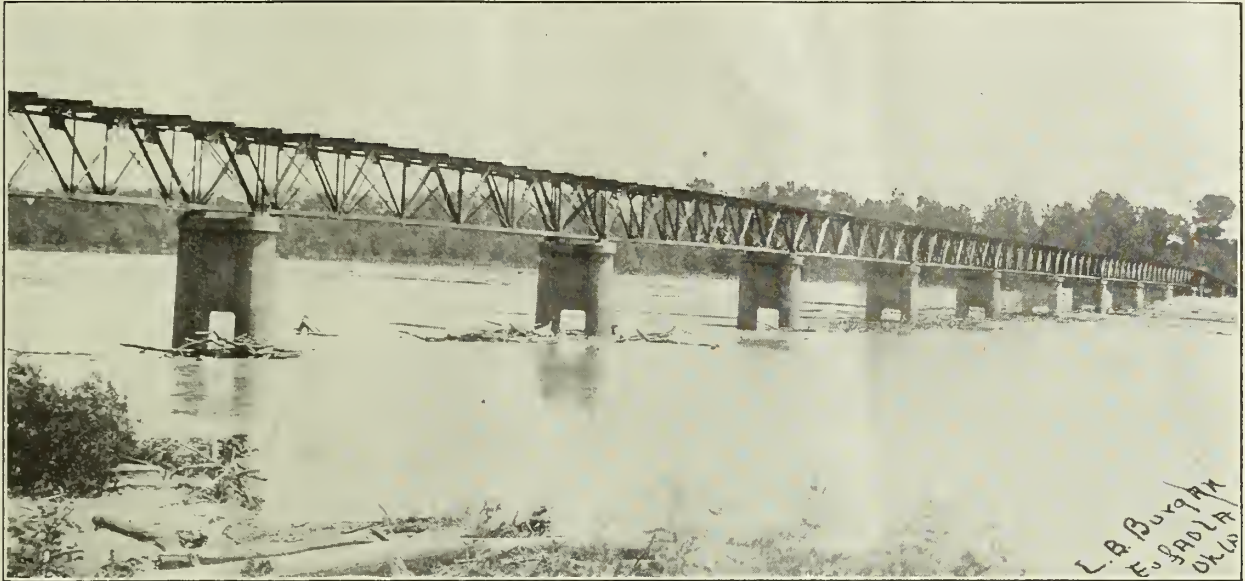
The New Canadian River Bridge
