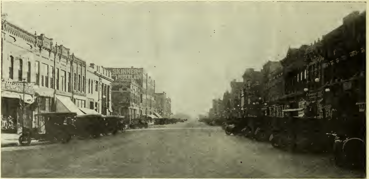
The course of the Jefferson Highway through Albert Lea, the metropolis of Southern Minnesota.
