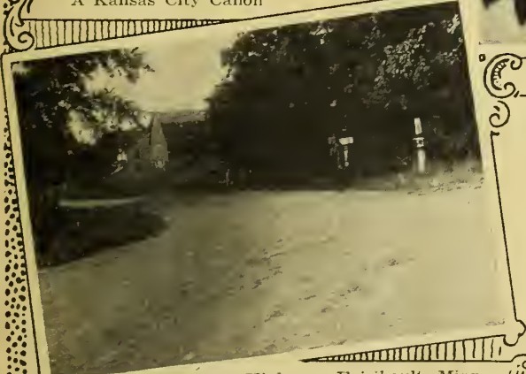
Jefferson Highway, Fairibault, Minn.
