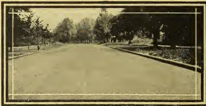
LONGWOOD DRIVE, CHICAGO Stanolind Paving Asphalt was used in building this splendid Asphalt-Macadam Road.
