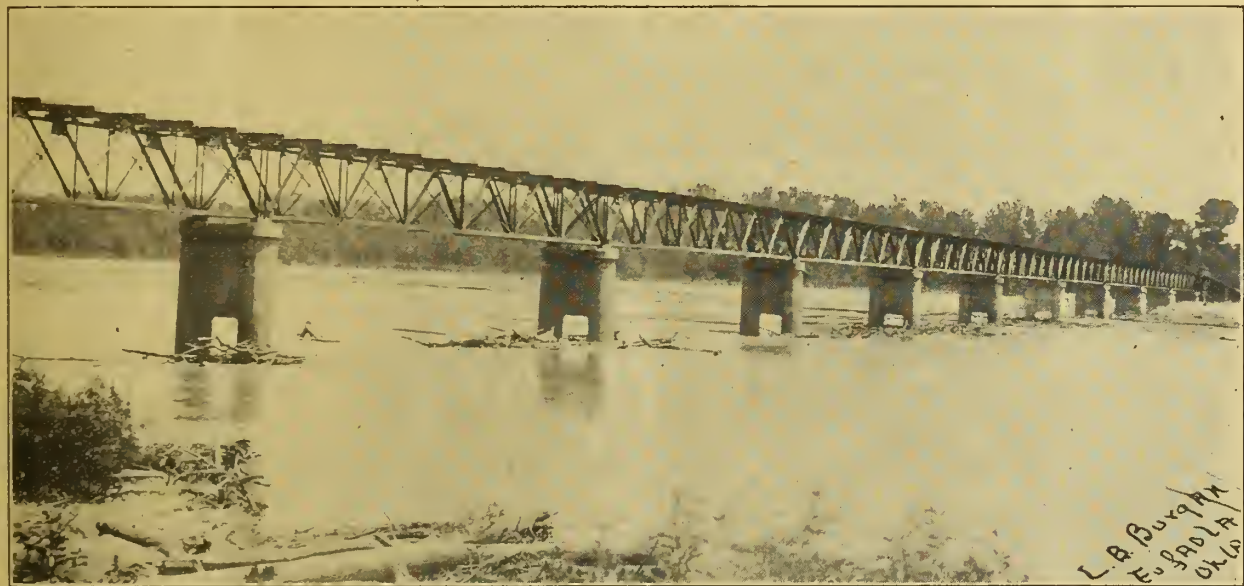
The Jefferson Highway bridge across the Canadian River, which will be open to travel this Fall.
