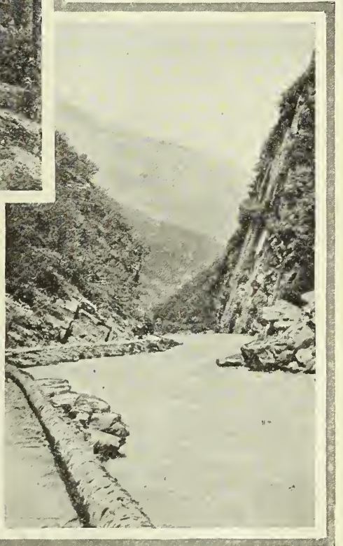
3. Keystone Canyon, showing how Valdez-Fairbanks Trail is re-enforced against Lowe River.
