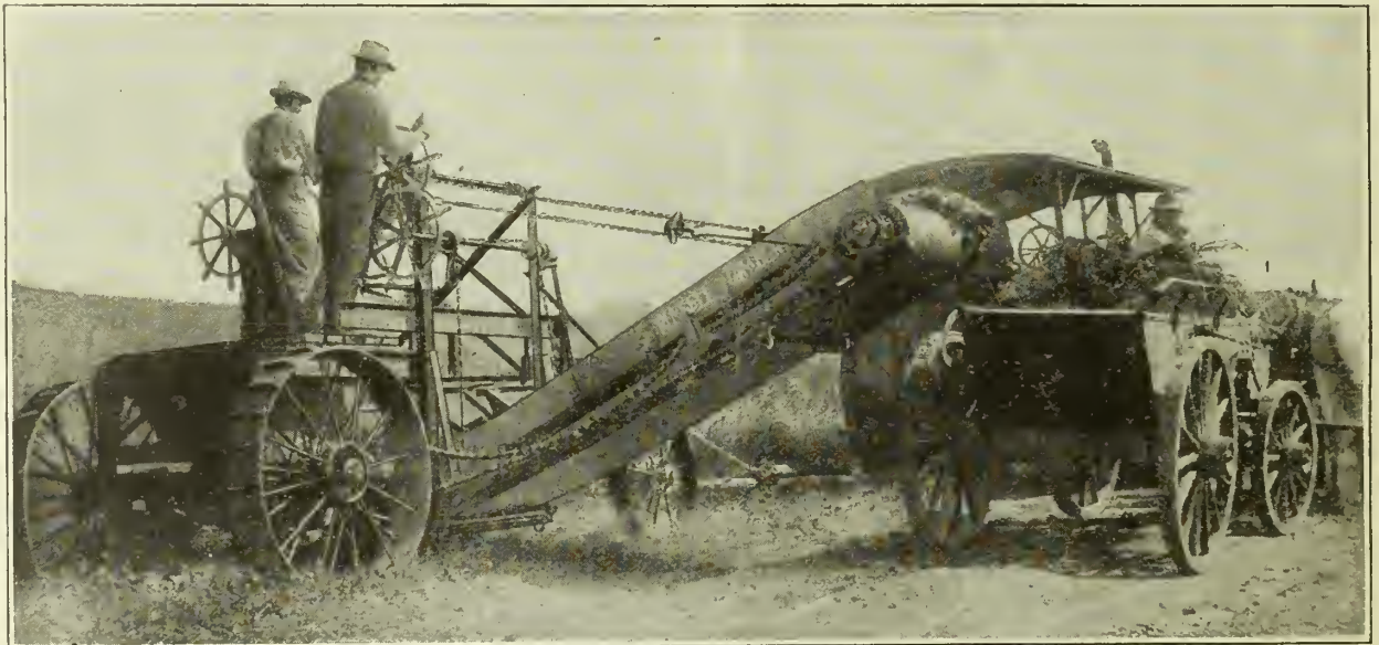
THE RUSSELL ELEVATING GRADER LOADING A RUSSELL DUMP WAGON
