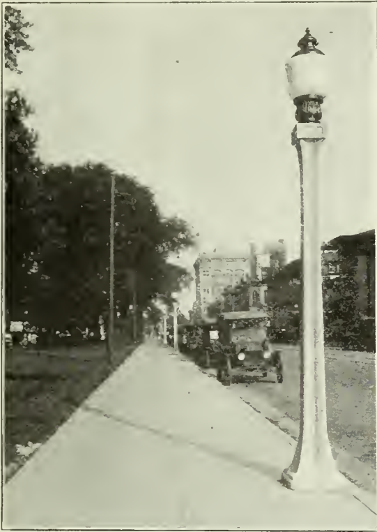
New Concrete Lighting Standards. West State Street, Mason City, Iowa.
