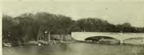
Where Cedar Falls, Iowa, will build her Auto Tourist Camp as a result of experience of H. F. McDougal on J. H.
