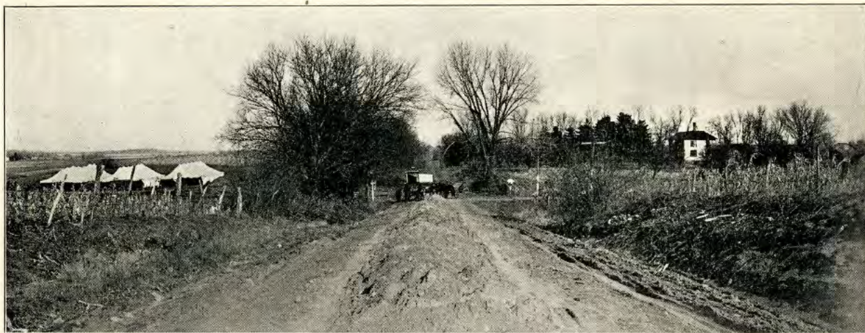
Putting gravel on the Jefferson Highway in Story county, Iowa. Note drift in center of road. When Mr. Ed Aldeman, of Nevada, in Story county, Iowa, promised Mr. Harry H. Polk, of Des Moines, Vice-President of Jefferson Highway for Iowa, to gravel the Jefferson Highway through Story county in 1916 every one thought he had promised the impossible, yet it has been done.
