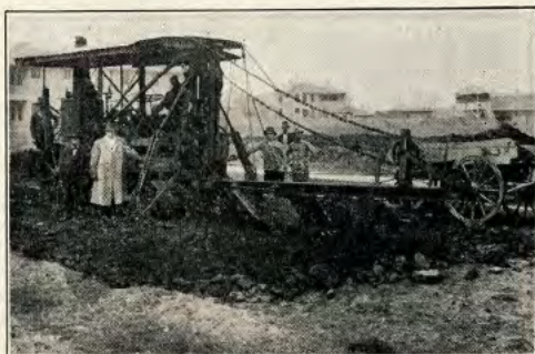
Road grading with "Skimmer Scoop," Rochester, New York.
