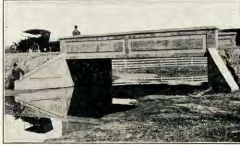
Thirty foot concrete bridge on Jefferson Highway in Caddo Parish, Louisiana, twenty miles from Shreveport.
