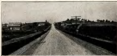
This trap rock macadam road, built eleven years ago, has never been resurfaced; it crosses the Jefferson Highway at St. Paul, Minn.
