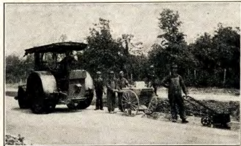
Ten miles of bitulithic pavement on Jefferson Highway from Winnipeg on road to Emerson.
