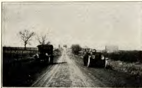
One of the contesting roads for the Jefferson Highway near Lamoni, Iowa.
