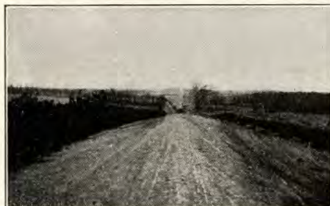
Widening the Jefferson Highway near Lamoni, Iowa
