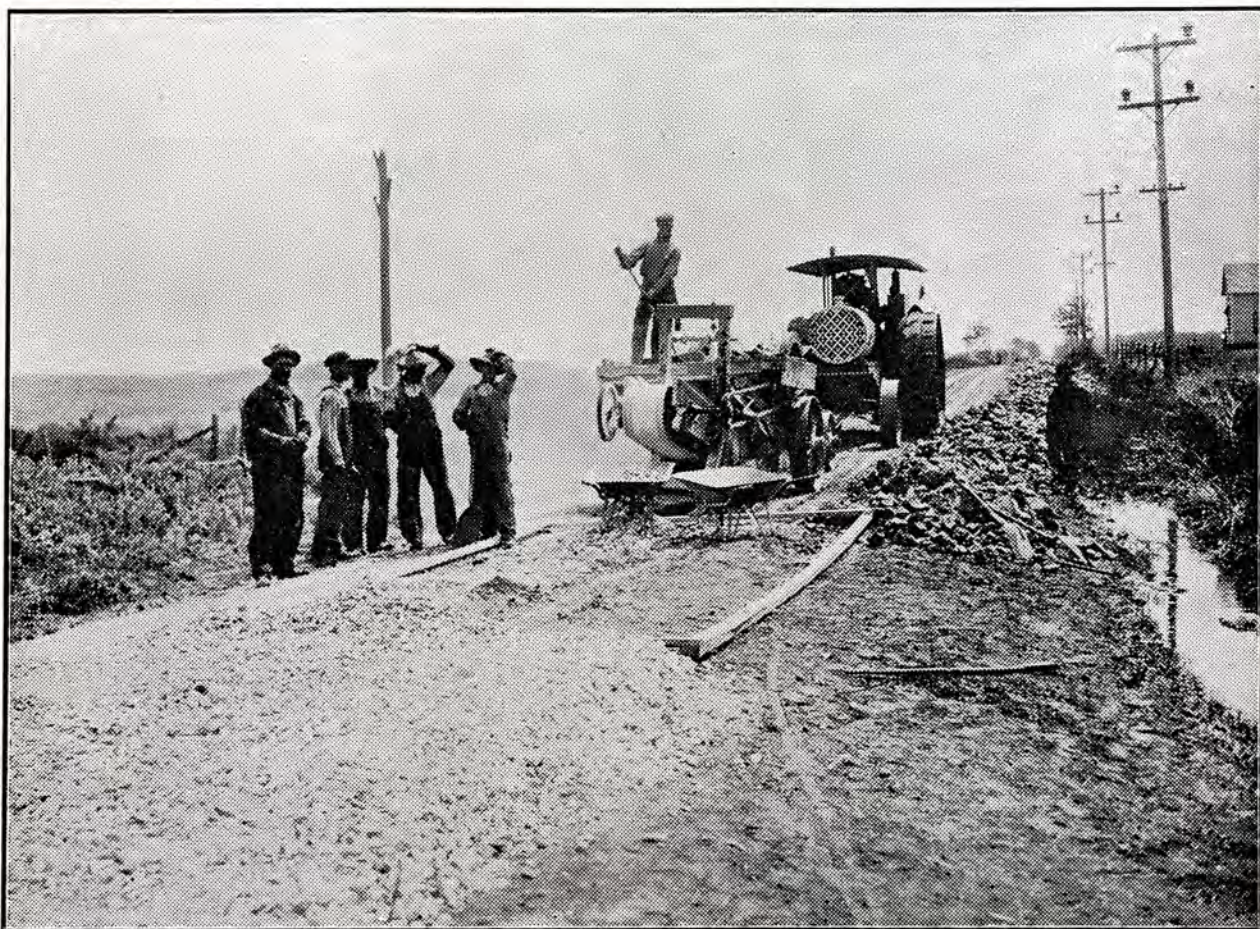
A "United" Portable Plant in Operation Crushing Material for Good Roads in Southwest Missouri.
