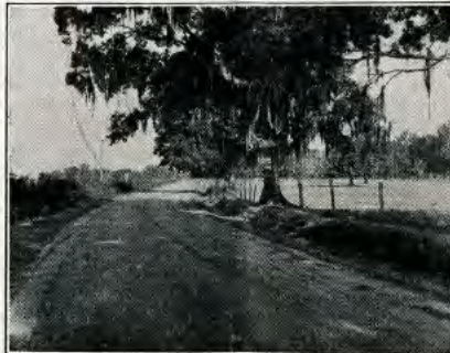
Concrete Surface on Jefferson Highway on Baton Rouge-New Orleans Section
