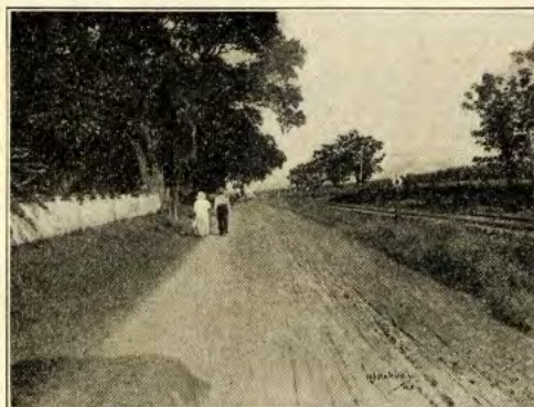
Good Roads, St. Bernard Parish, La.
