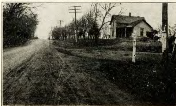
Section of Inter-State Trail at Iowa Falls, Iowa, a part of the Jefferson Highway. This view was taken to show marking post which appears at right of picture. The Inter-State Trail is well marked from St. Paul to Kansas City.
