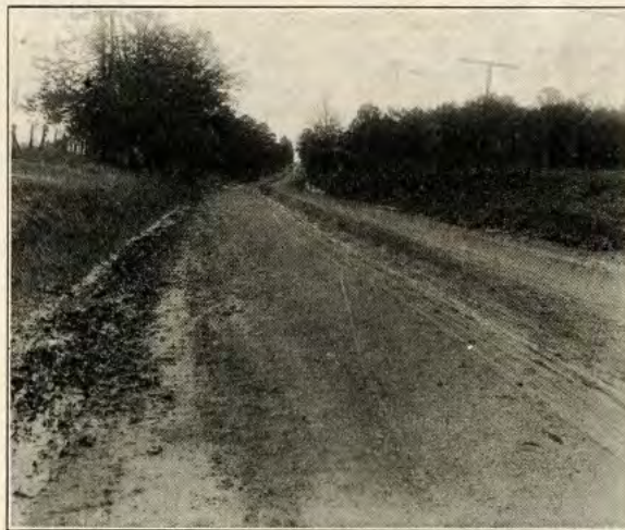
Section of Jefferson Highway near Marshall, Texas.
