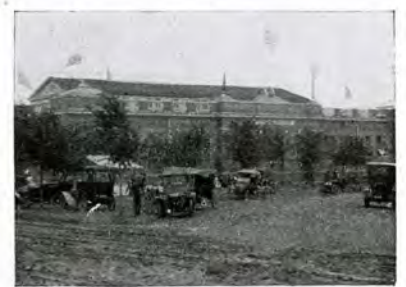
The Dairy Building
