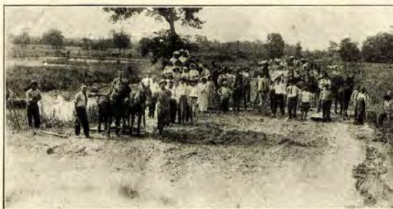
Volunteers repairing levee at Sulphur Springs, Texas.
